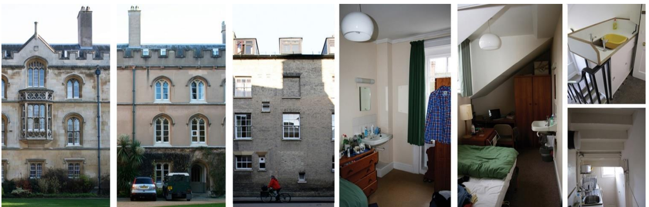
Figure 2. The existing building. Externally the River, Court and rear facades are finished with different materials, of differing quality and character and characteristics of vapour and moisture resistance and permeability. Internally the spaces illustrate a history of iterative interventions, replannings and the ad hoc installation of services and amenities.
