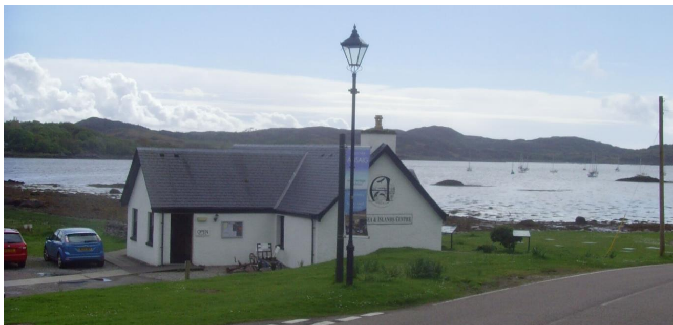
Figure 1. View of LSIC building, north facing entrance and reception and north gable wall of exhibition area.
