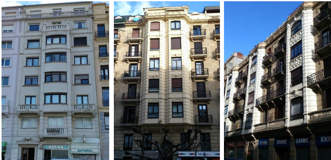
Figure 3. Buildings of built heritage of Gros District that requested license for energy rehabilitation. Zurriola 22, Colon 17 y Usandizaga 3. Source: Author.
