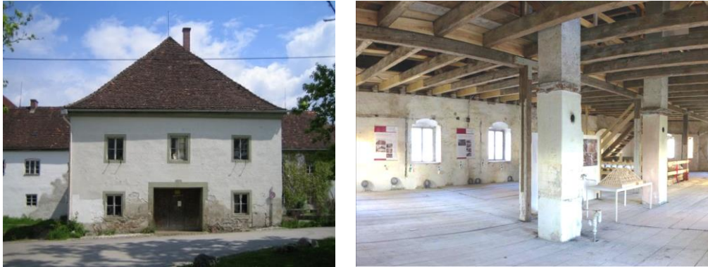
Figure 1. The “Alte Schäfllerei” in Benediktbeuern monastery accommodates the Fraunhofer Centre for Conservation and Energy Performance of Historic Buildings (left). On the upper floor innovative insulation materials are reversibly applied and their hygrothermal performance is examined (right).
