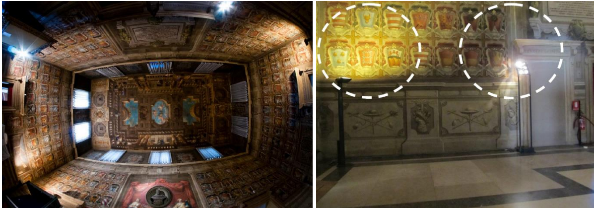
Figure 3. Left: View from below of Sala Urbana’s frescoed ceiling and walls. [7] Right: Pre-3ENCULT - the lighting system produces high inhomogeneity and glare. [6]
