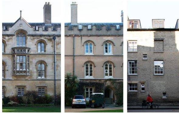
Figure 1. The River, Courtyard and rear facades are finished with different materials, with differing characters related to their urban significance and differing characteristics of vapour and moisture resistance and permeability.
