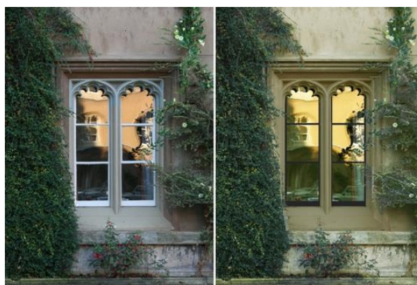
Figure 5. Before / after images of the treatment of windows and external render. The colour of the render and cast-iron window traceries and the dark colour of the window frames reinstate the integrity of the gothic 'pierced' wall plane.
